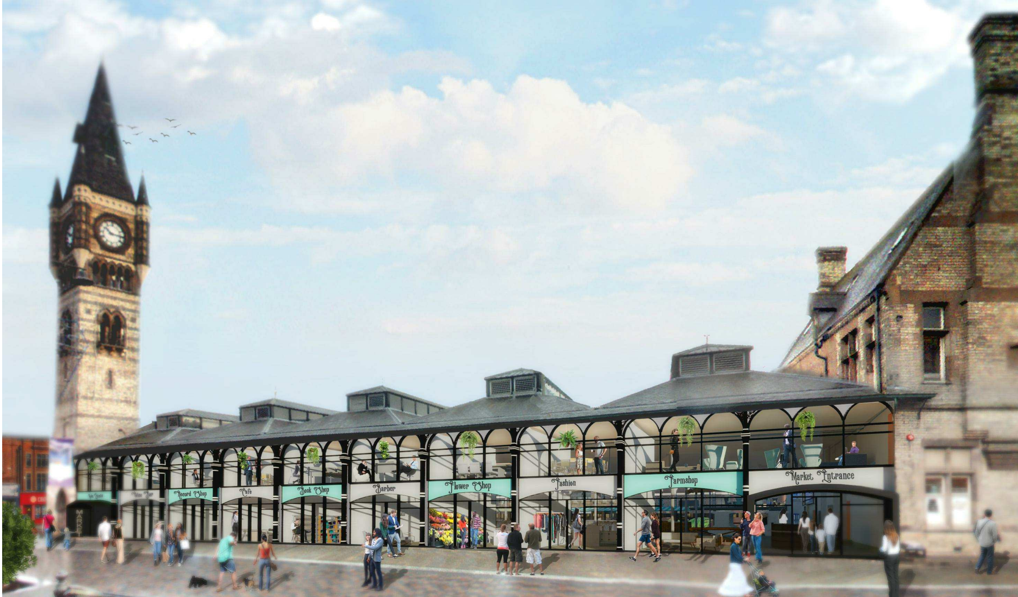
Exterior - West Row
